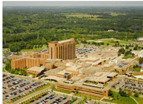
Saint Joseph-Mercy's sprawling Ann Arbor campus: In the midst of a building boom that added half a million square feet, the system realized over $2 million in energy savings.
